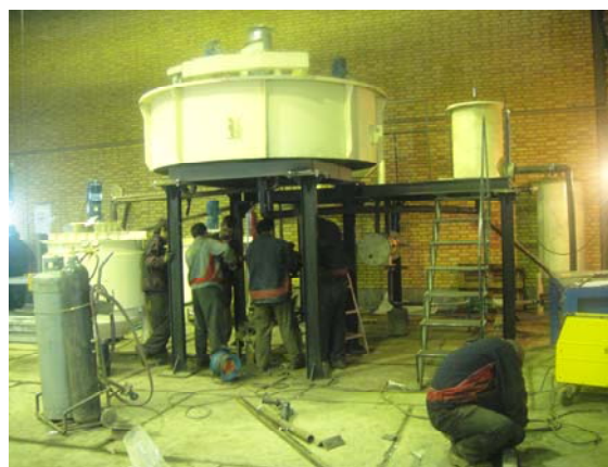
Fig.4. Assemblage process of pilot system
