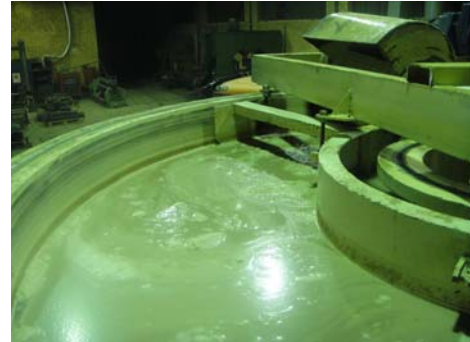
Fig.7. Floatation tank of pilot system after starting the system
