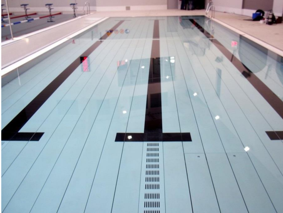
Figure 12: Moveable swimming pool floor (source: Variopool)
